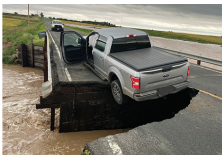
A bridge failure from the flooding on 144th – and the consequences of violating the barricade.
